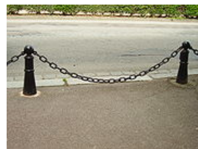
Figure 7.1: A hanging chain forms a catenary. http://en.wikipedia.org/wiki/Catenary
